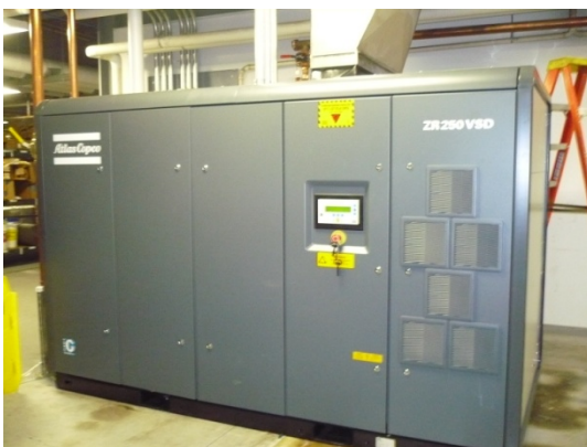
350 hp water cooled air compressor
