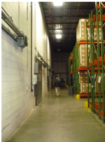
High Output T5 Fixtures with occupancy sensors
