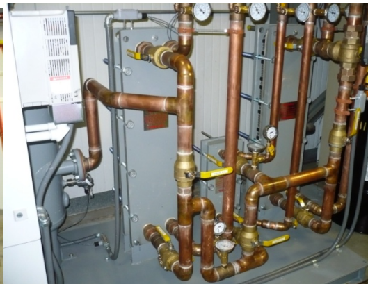
Hot water recovery system
