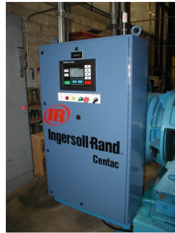
New air compressor control cabinet
