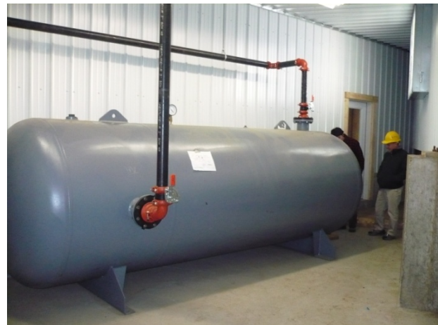
2,120 gallon air receiver (compressed air storage tank)
